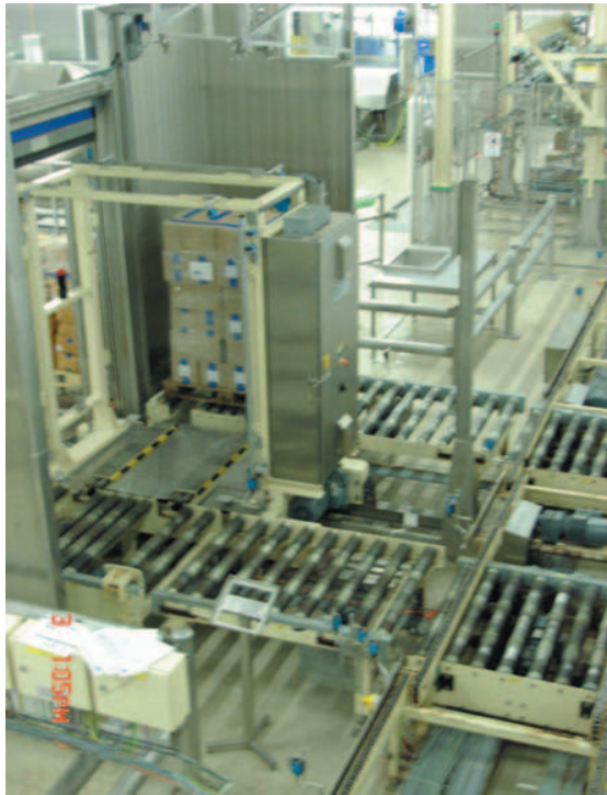
Goods recovered from the store for the first time are transferred to in-house pallets on the upper level. After pallet transfer the goods are taken by transverse transporters to the consignment workplaces.
