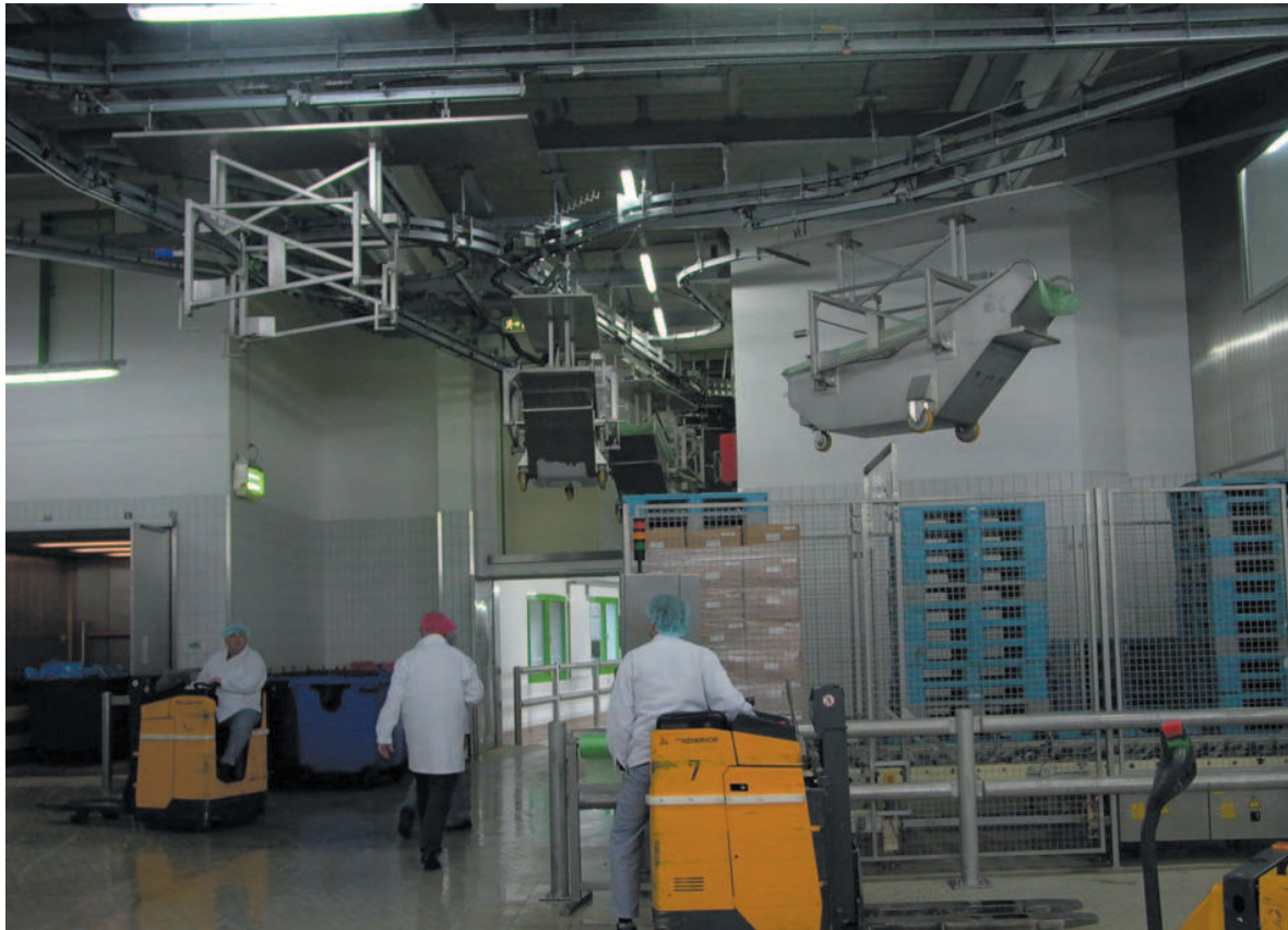
Full transport containers are transferred by a hoist to the overhead conveyor, which automatically takes them from there for processing
